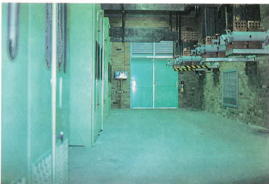
Fig. 4: Inside the rectifier building. On the left are the diode cubicles. The DC busbars are on the right. Some of the copper busbars are visible at the top.
