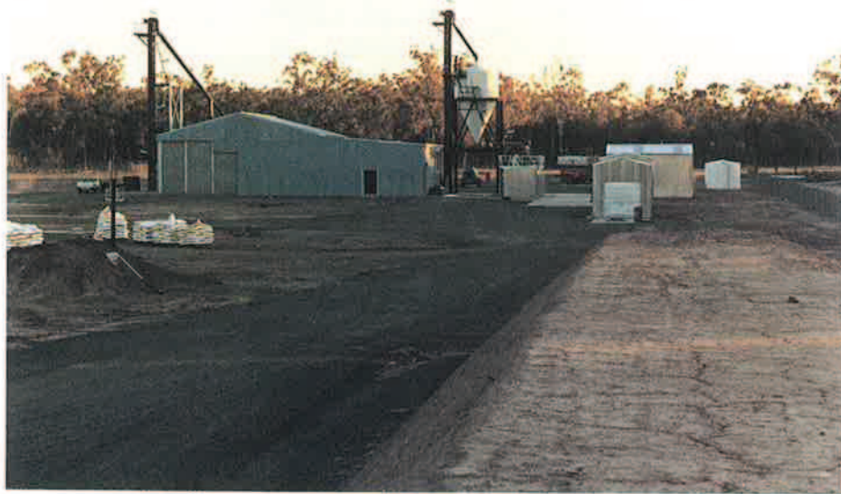
Fig. 3: 400-tonne capacity bulk ammonium nitrate storage shed erected at German Creek mine in central Queensland. This facility and associated equipment is designed to supply bulk ANFO and bulk Watergel explosives to the German Creek mine.
